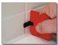
If necessary, use FUGI II with guiding aid to assist you in crossing grout joints.
