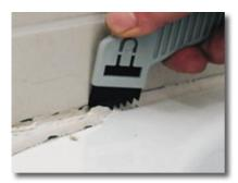
Remove old caulking with saw blade. Whatever is left on tiles or other smooth surfaces can be removed with the scraping blade.
