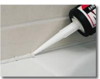
Apply the caulking mass. Since there is no need for a releasing agent, just work step-by-step, by only doing short distances.
