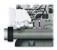
Disconnect heater output by removing two screws at the bottom of circuit board. Disconnect pressure switch.
