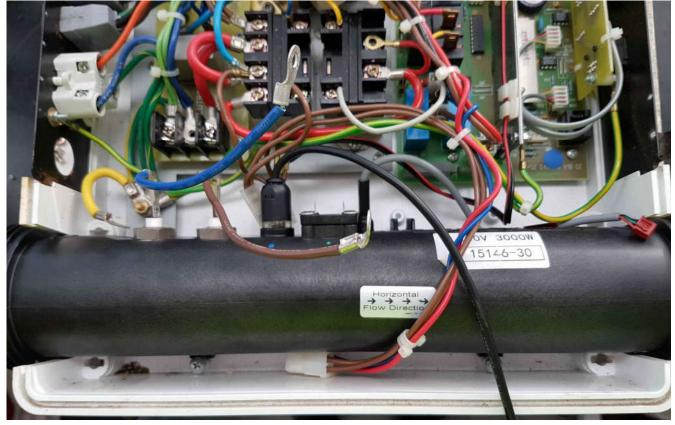
12. Remove the new element earth screw and place the earth wire onto the new element and secure it with the screw. Make sure that the earth wire is coming from the left hand side of the controller and is parallel to the heater tube; otherwise you will not be able to sit the element in the correct position later on.
