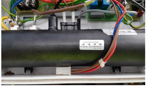
15. Connect new element blue neutral wire to screw terminal block and secure it with the screw.
