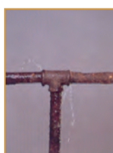
Leaking Joint
